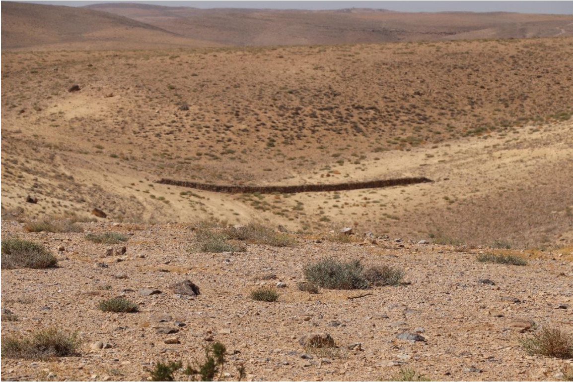
Figure 20: Water Harvesting Structures in Al Mansheyyeh Range Reserve
